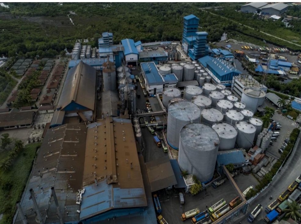
GAR's oleochemical plant in Medan PHOTO: NANANG SUJANA
