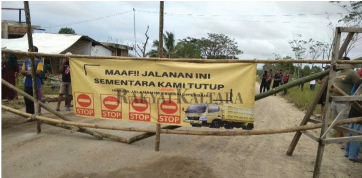
Figure 31. Road closure sign near the Phoenix mill construction site in Tarakan.
